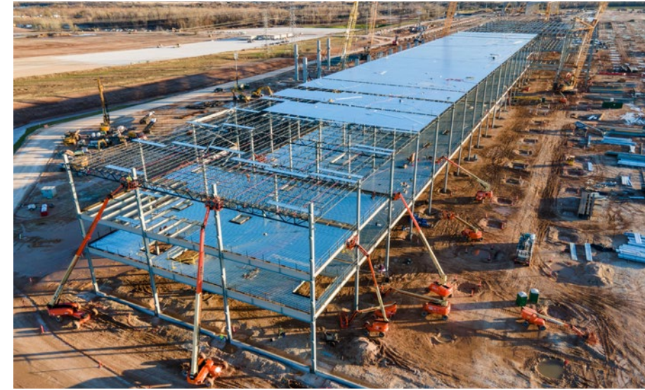
Tesla gigafactory construction in Austin, TX
